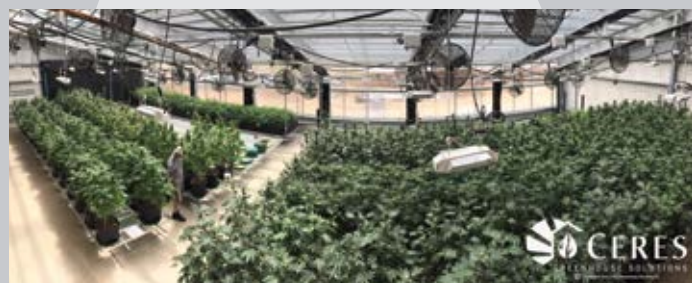
Hybrid Greenhouses- up to 96% light transmittance with ETFE Glazing
